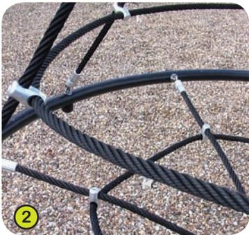
2- **The Polyfix rope**,  $\varnothing$  16 mm, is made up of six,  $\varnothing$  0.8 mm, galvanised steel cables. The rope is covered with polypropylene.
