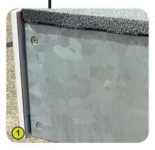
1- The framework is made from hot-dip galvanised steel.
