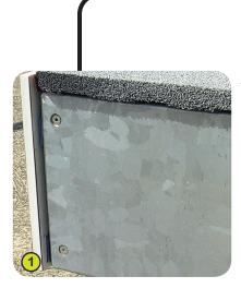
1- The framework is made from hot-dip galvanised steel.
