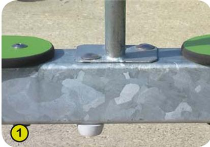
1- **The 90x90mm square tubes** are made of galvanised steel, ensuring robustness and durability of the equipment.
