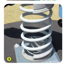
**5- The stainless steel fixings** are protected by polyamide anti-vandalism caps.
