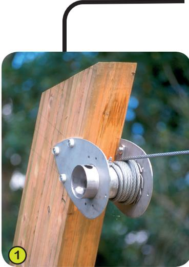
1- **The shaped cableway beams** are made of oven-cured laminated wood with a surface coating; they are 95mm thick, 200mm wide, and 3.2m high, and they give the structure considerable strength. They are anchored in metal sleeves. The cable tensioning system has a pawl which allows easy tensioning of the 10mm diameter galvanised steel cable.
