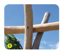
**1- The posts and the horizontal beam** (diameter 120 to 140mm), are made from sap free robinia.
