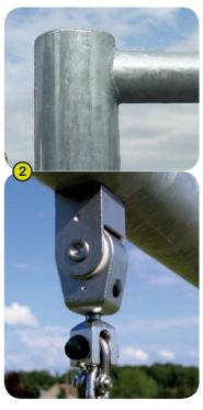
The horizontal beam of the swing is made of non-painted galvanised steel.
