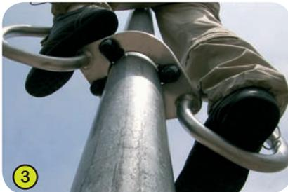
3- The **climbing system** (feet) is made of stainless steel.
