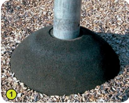
1- The **rubber pad** is located at the base of a mast made of galvanized steel.
