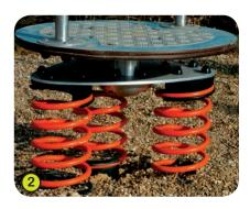
**2-** The oscillation system is based on the interaction of three highly resistant steel springs (35SCD6 grade steel) fitted with anti-trap retention components (patented by Proludic).
