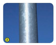
2- The 90mm diameter post is made of galvanised steel.
