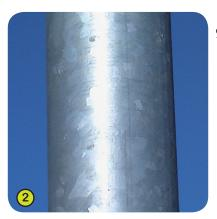
2- The 114,3mm diameter post is made of galvanised steel.
