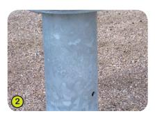
2- The 90mm diameter post is made of galvanised steel.
