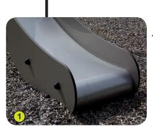
1- The sliding surface and the platform are made of stainless steel 2mm thick, which are shaped, bent and rolled from one piece.
